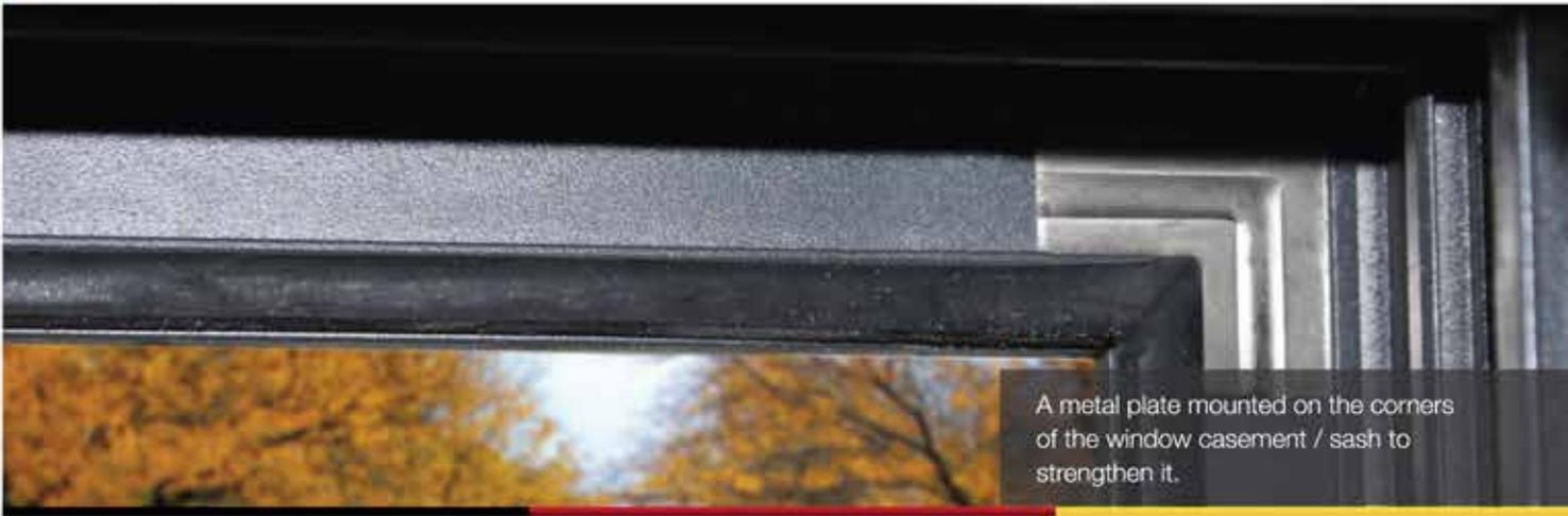
A metal plate mounted on the corners of the window casement / sash to strengthen it.
